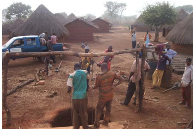
HAND DUG WELL INSTALLATION IN REMOTE FULBE REFUGEE VILLAGE
