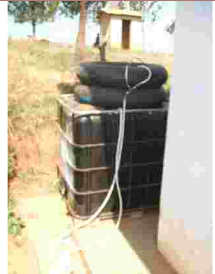
Our biogas demonstration produces methane to heat tea for visitors.
