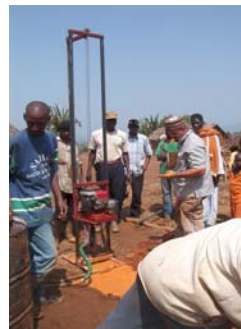
Test drilling in village
